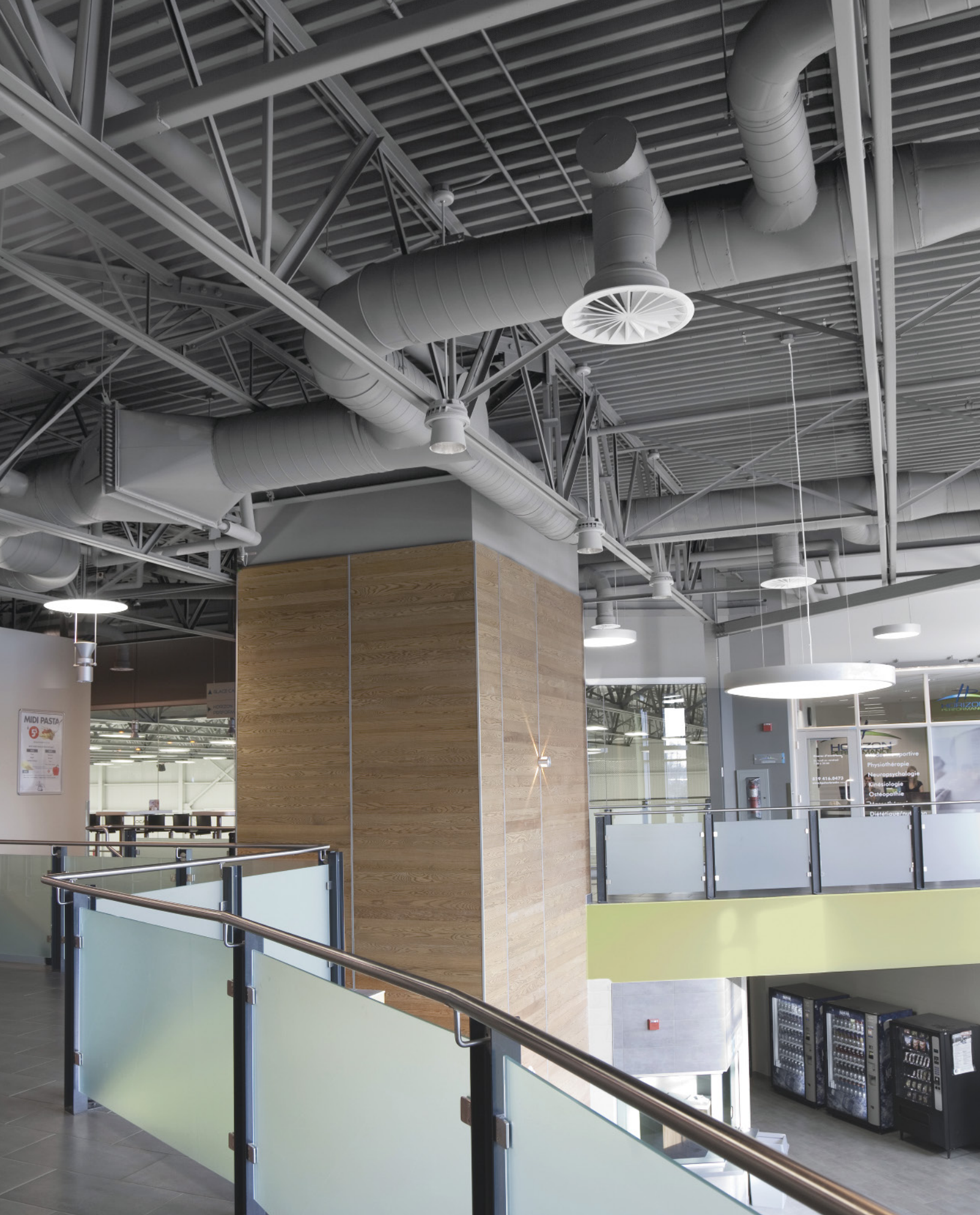
DRS diffuser, Thibault/GM Sports complex, Sherbrooke, Canada
