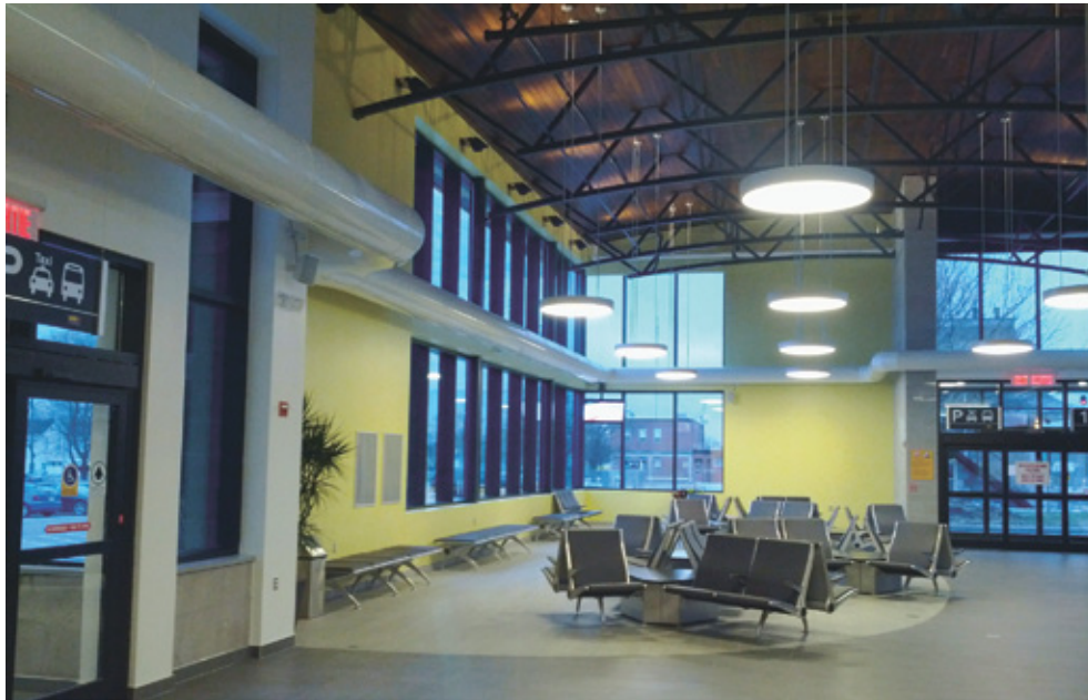
RRA Duct diffuser
